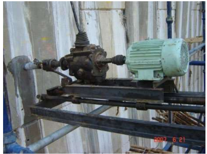
Fig. 4 : The drilling operation for installation of soil nail
