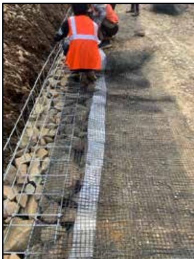
Fig. 10 : Welded wire mesh unit connection with geogrid and 600 mm drainage layer for reinforced soil walls at Shimla Bypass Project
