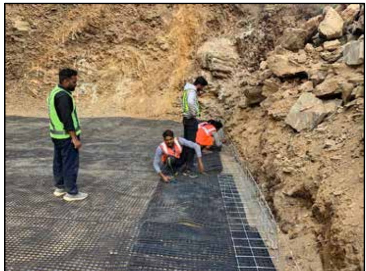
Fig. 10 : Welded wire mesh unit connection with geogrid and 600 mm drainage layer for reinforced soil walls at Shimla Bypass Project
