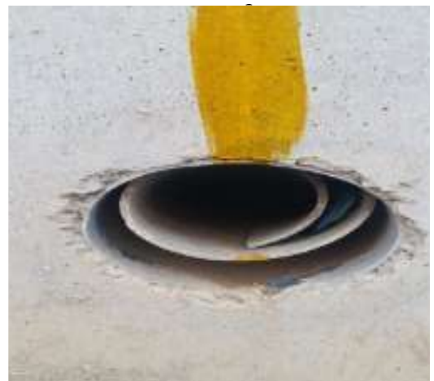
(j) Drainage hole condition
