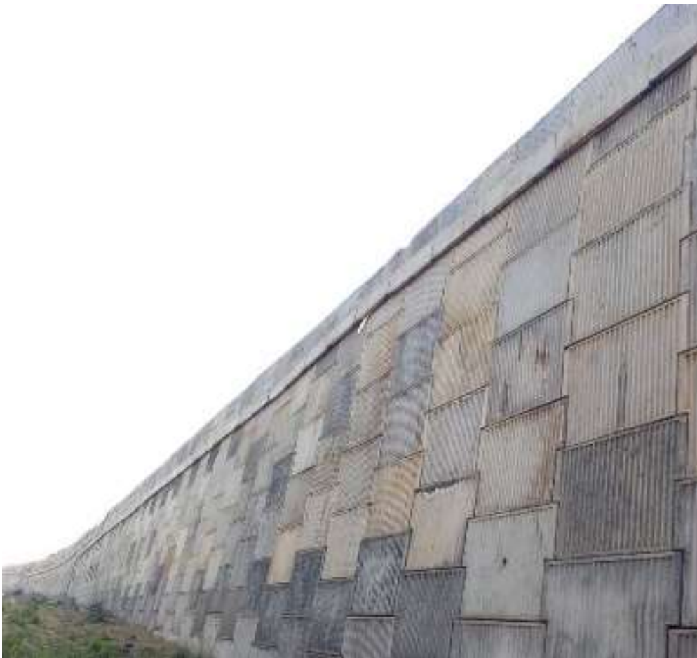
Fig. 9 : Site photograph of completed structure
