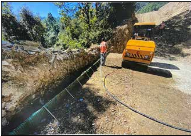
Fig. 9 : Welded wire mesh unit along with wraparound geogrid and coir erosion blanket for reinforced soil slopes at Shimla Bypass Project
