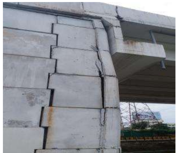
(f) Dirt wall, Abutment edge and RS wall panel condition
