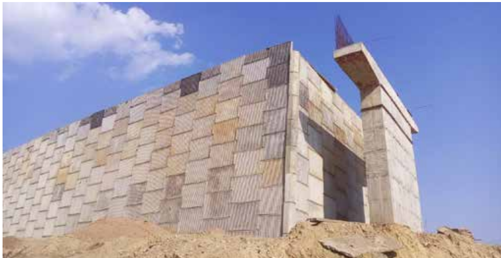
Fig. 6 : Site photograph of RSW on LHS side of Bimalgarh ROB
