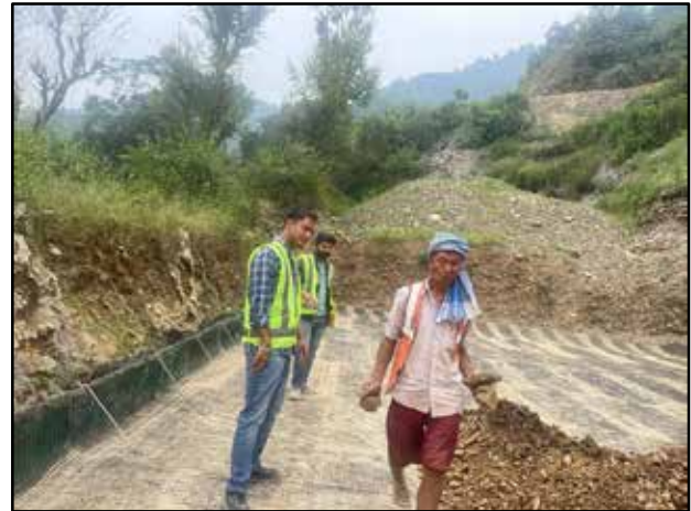
Fig. 9 : Welded wire mesh unit along with wraparound geogrid and coir erosion blanket for reinforced soil slopes at Shimla Bypass Project
