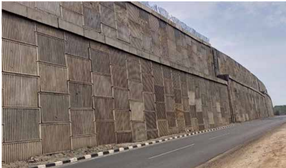
Fig. 7 : Site photograph of RSW on RHS side of Bimalgarh ROB
